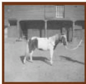
Coachman's House South Facade in 1897.
